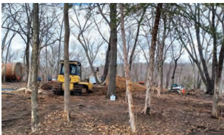
Clearing out top track/spectator area and installing water tanks.
