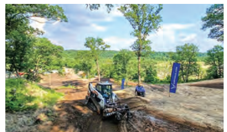
Upper track Maintenance.
