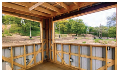
Early construction of Score Shack.
