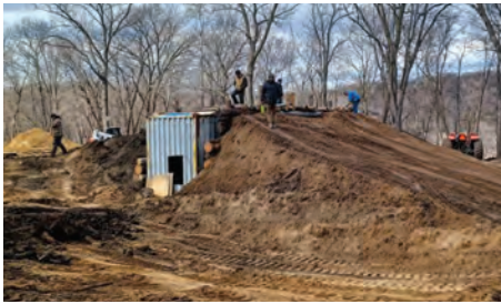
Early installment of tunnel jump.
